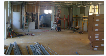
MorningStar Renewal Center Renovation in progress, 2008 · Pinecrest
