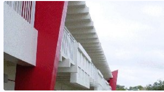
Monsignor Edward Pace High School Classroom building · Miami Gardens
